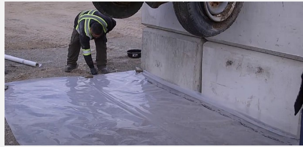
Figure 10. Polyethylene sheet under an elevated ELV
