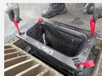
Figure 3: LittaTrap™ Source: https://www.enviroprod.com/products/littatrap
