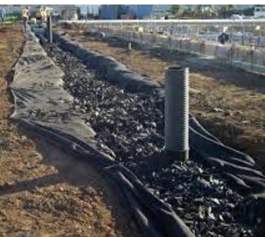
Figure 8: ELT replacing gravel in LFG extraction well
