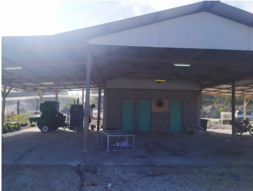
Figure 1: Waste segregation building at the waste facility
